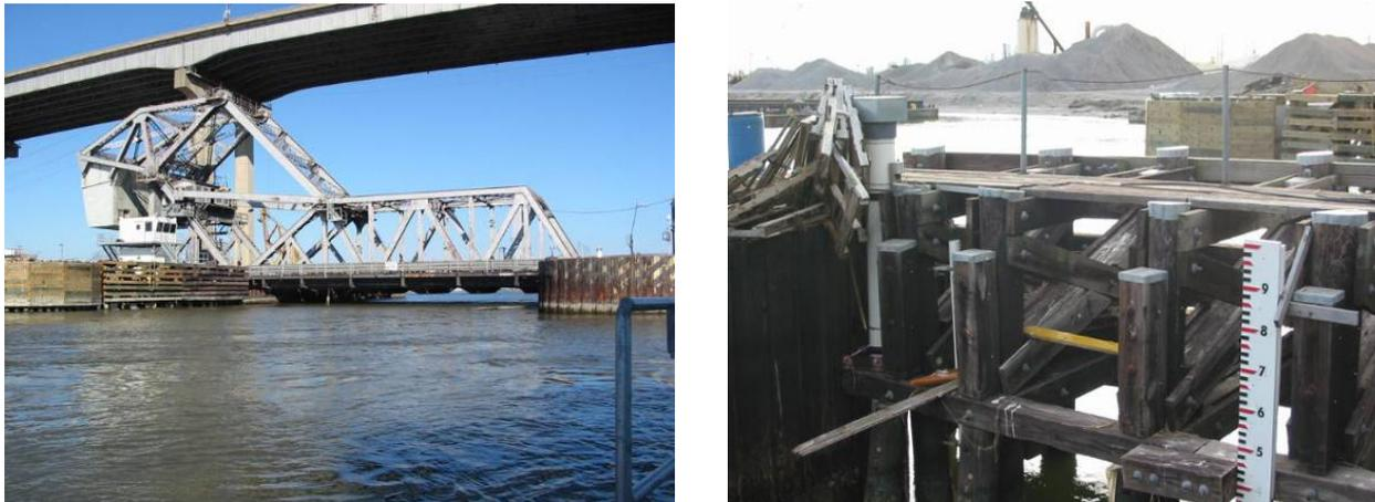
Figure 64. (Left) IHNC Almonaster Bridge—low chord elevation 3.51 ft NAVD88 (2004.65). (Right) Leveling to USGS recording gauge and Orleans Levee District staff gauge on I-10 bridge over IHNC.
